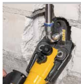
REMS pressing ring 45° (PR-2B) Patent EP 2 774 725
